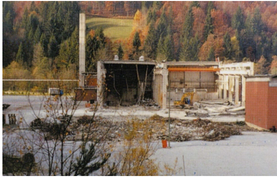
Figure 8. Dismantling of the processing plant
