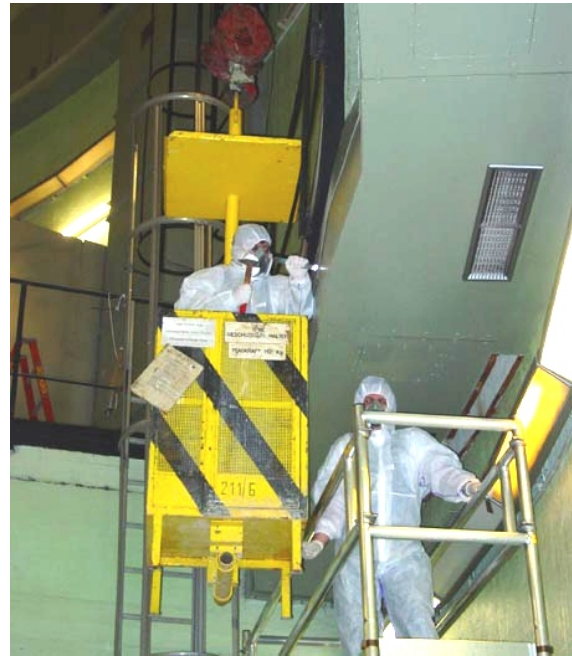
Figure 1. Dismantling of the ventilation system
