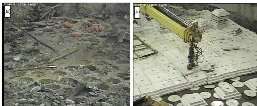
concrete slabs and blocks. All the slabs and containers were loaded onto the trolley and transferred to the SRW module where they were checked with dosimeters, separated into low- and intermediate-level waste, marked, wrapped in polyethylene film, and moved out of the site. They were then loaded onto trucks and transferred to the storage areas.
