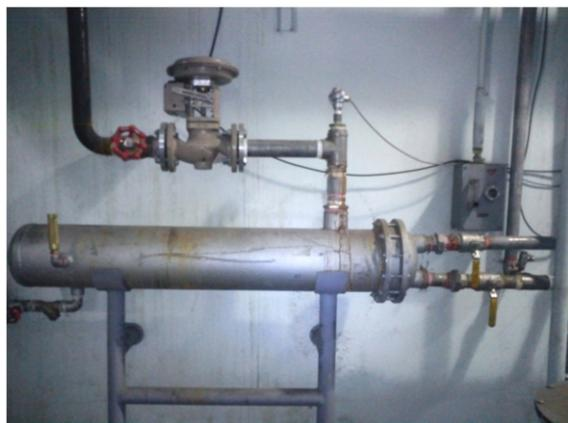
**Figure 4.** HWLS, as installed in the HVAC room and connecting pipes
